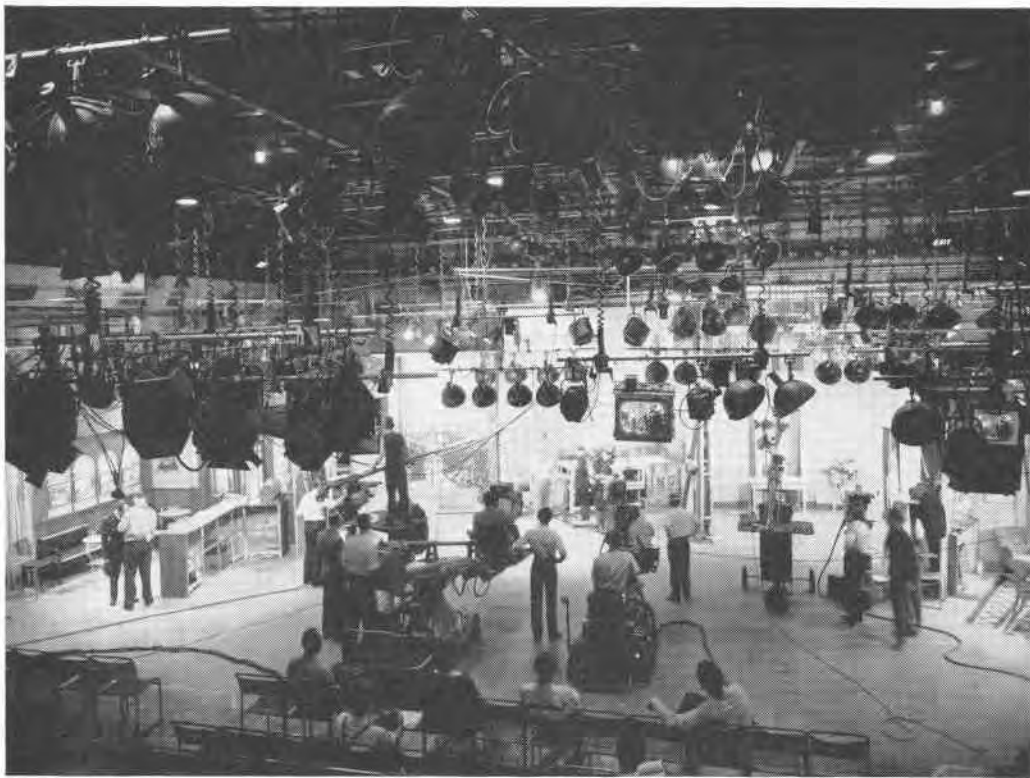
A rehearsal in progress in one of the BBC's most modern studios at Riverside, Hammersmith. The lighting battens, which can be raised or lowered electrically from a control desk on the studio floor, are clearly shown. The switching and dimming of the illuminators, individually or in groups, is performed by remote control from a lighting console adjacent to the Vision Control Room.
