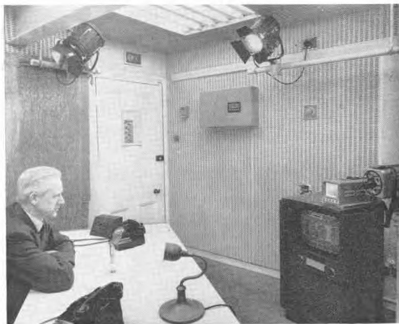
The BBC's first unattended television studio at St. Stephen's House: showing the small photoconductive - type camera and its monitor on which the Correspondent can check that his picture is satisfactory, a television set for checking the picture transmitted from the Crystal Palace television station, working and spare microphones, and fixed lighting.
