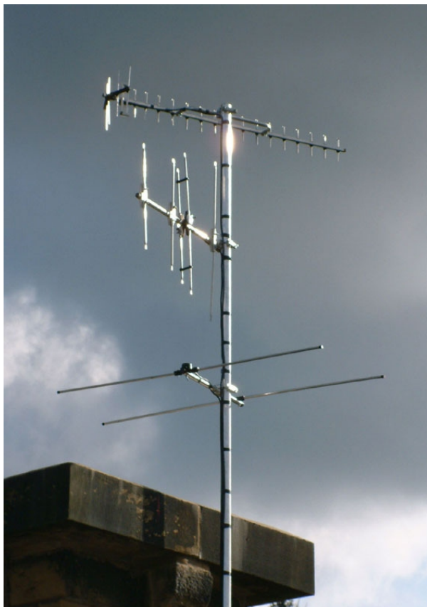
Fig 4. Good clean incoming signals are the essential starting point for every system. From top to bottom: Vertically polarised UHF TV aerial, four element VHF DAB aerial, two element VHF FM aerial.
