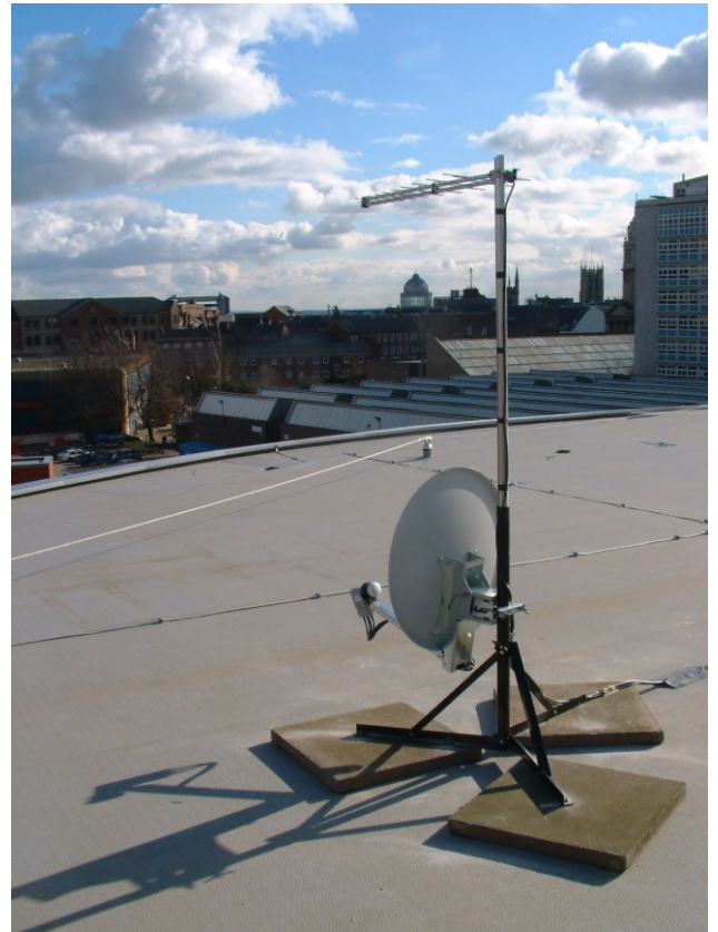
Fig 15. This 65cm dish and log-periodic UHF aerial are fixed onto a steel groundstand. The groundstand is bolted to three concrete slabs and these stand on rubber sheeting to protect the roof membrane.
