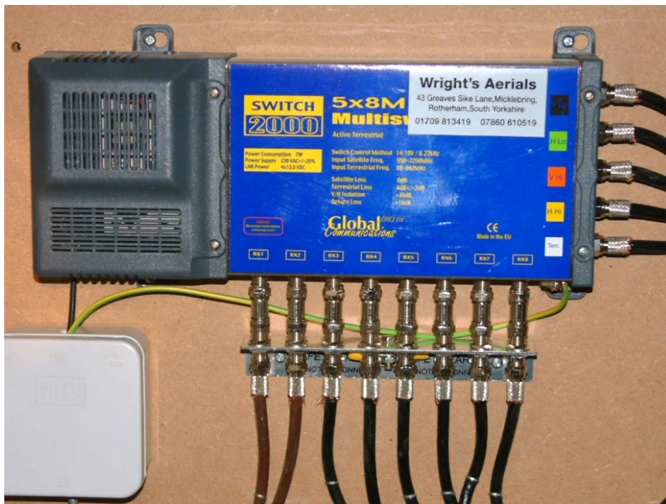
Fig 3. Global 5x8M mains-powered multiswitch in situ. The one terrestrial and four satellite inputs are on the right, and the outputs are along the bottom. This photograph was taken before the installation was earth bonded.
