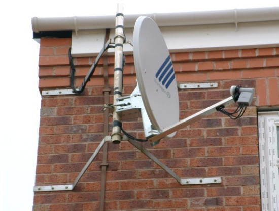
Fig 14. 75cm Hirschmann dish fixed on a pair of 600mm tripod stand-off brackets.
