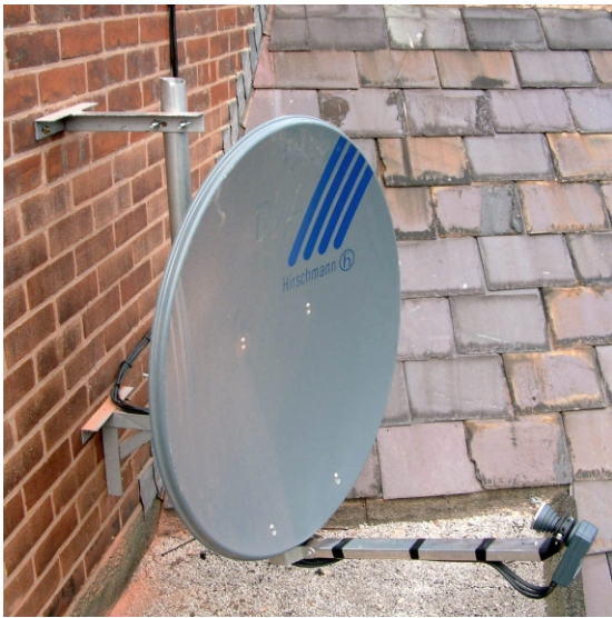
Fig 12. 65cm Hirschmann dish fixed on 'T & K' wall brackets.
