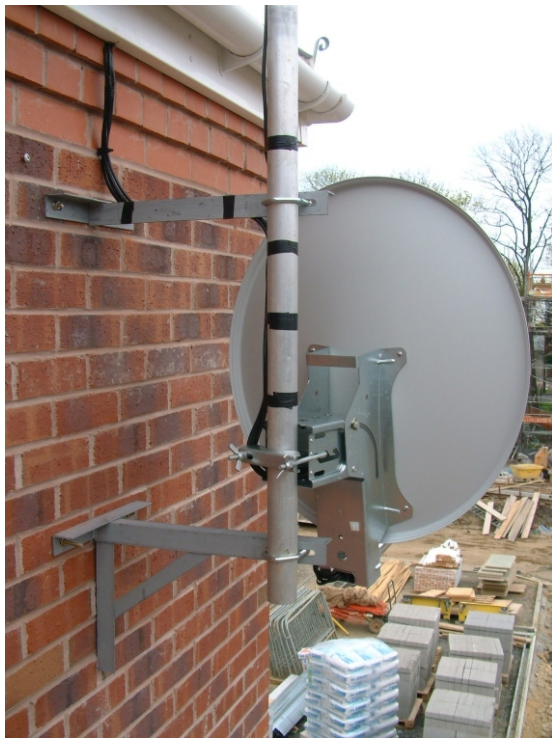
Fig 13. Another 65cm Hirschmann dish fixed on 'T & K' wall brackets.
