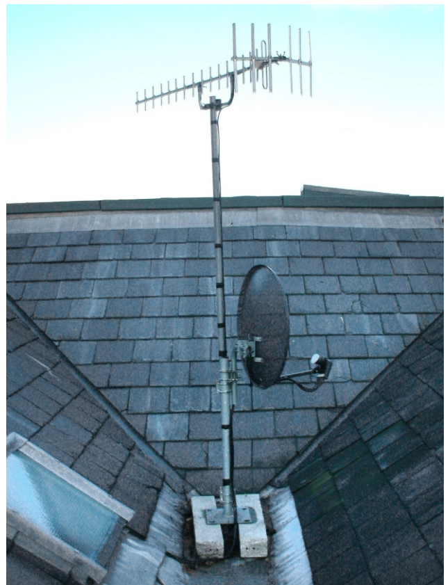
Fig 16. A groundstand with a small base and no diagonal supports has very little strength. It should only be used to support a very modest load and even then it needs to be bolted to a large piece of concrete, not to a pair of path edgings like this. It was possible to push this installation over with one finger!
