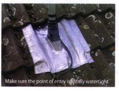
tile you are going to remove. This is roof work, so you must use a proper ladder, roof crawler, and safety harness, and take great care. Most tiles are easy to lift. They are usually held by one nail. A slate roof is different; unless you know what you're doing don't disturb slates or slate-effect composites.
