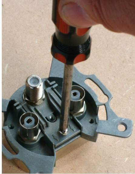
2 Unscrew the braid clamp.
