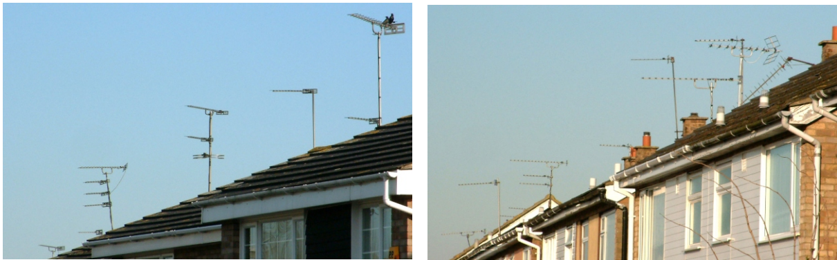
Fig 7.2.2. Typical aerials in Clacton. Every aerial is aligned on Sudbury. The older aerials are almost all Group B, whilst the new ones tend to be ‘high gain’ wideband types.
